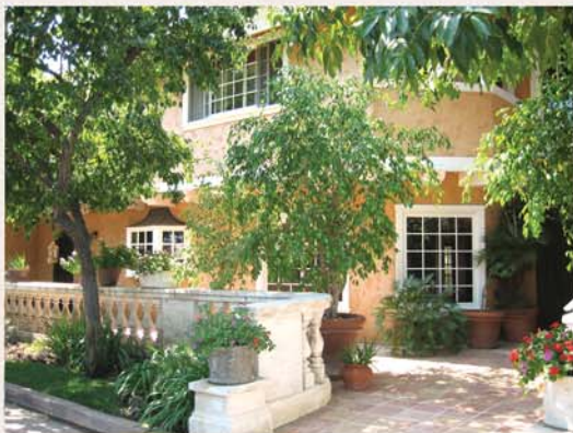
REFURBISHED: This Spanish home, owned by Nikki Sixx and Donna D'Errico, is on a 40-acre lot.
